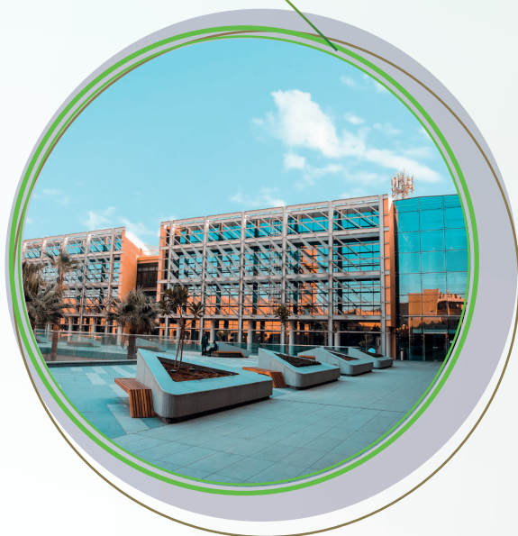
RCRC Expansion Project
