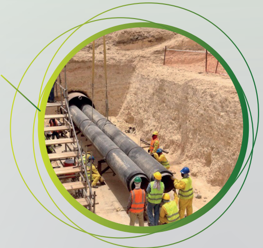
Ground Water Level Reducing, Riyadh.
